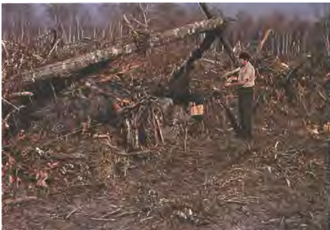
Dirt in windrows can aggravate smoke management problems
